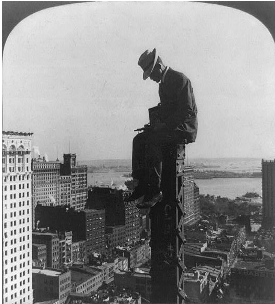
A dangerous position for a photojournalist reflecting some of the precarity faced by contemporary journalists who have to navigate media law, regulation and ethics. 'A dangerous position' by H.C. White Co. photographer working on column of new building, 250 ft. above ground, New York City in 1907. US Library of Congress.
